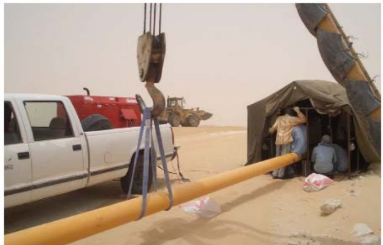
Oil pipeline construction
